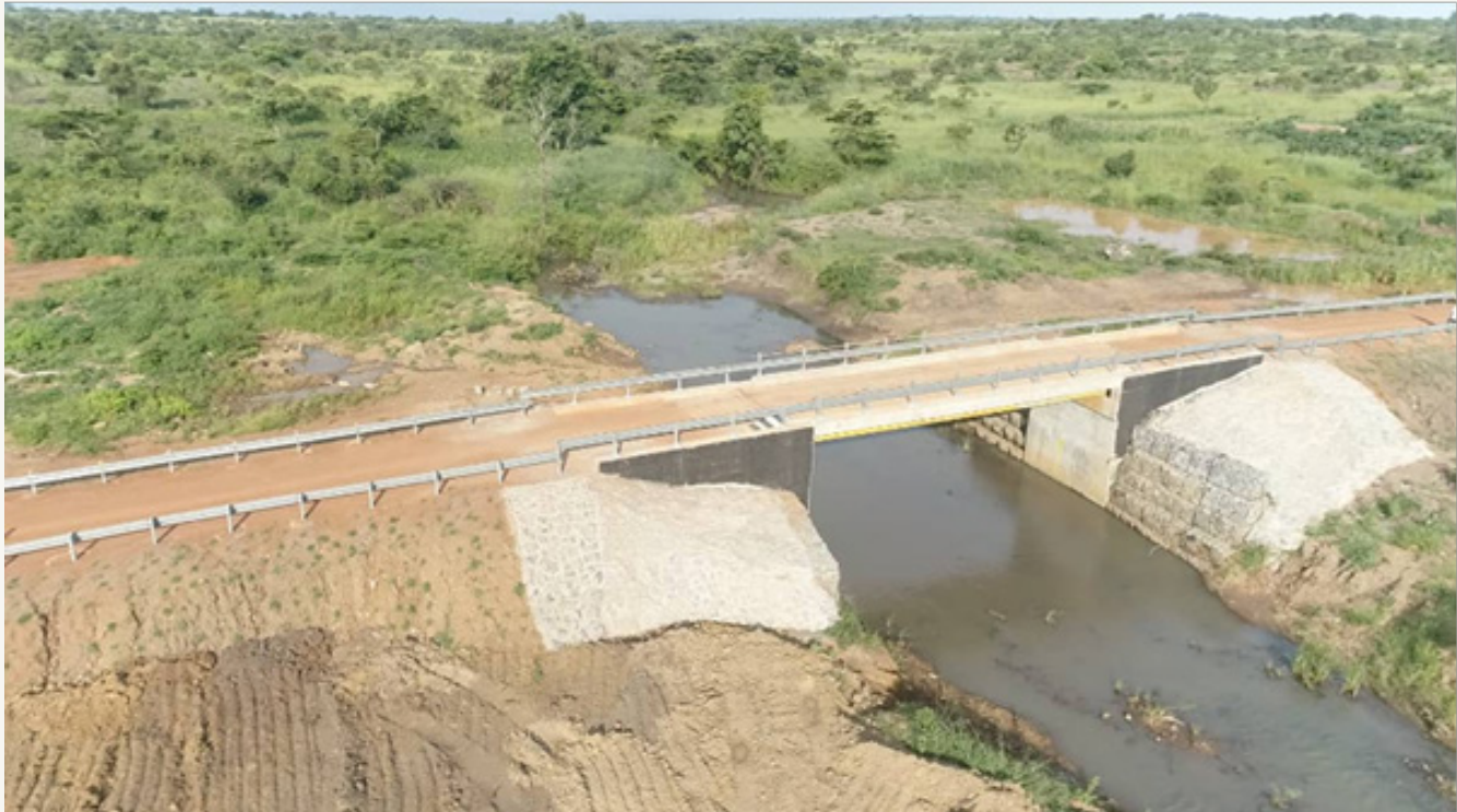
Lanyandang Bridge in Kitgum District -Constructed under NUDEIL
