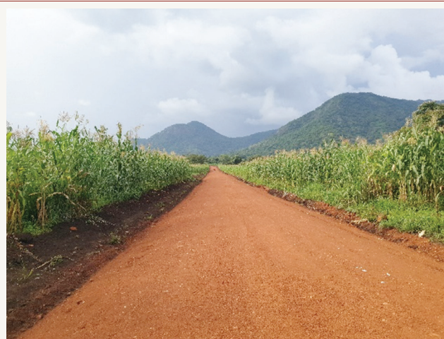
Olaya - Rukuk Community Access Road in Orom, Kitgum District
