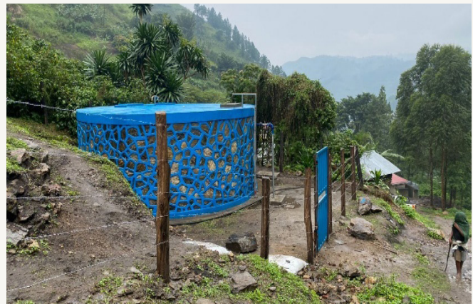
Left: Hon. MoSLG commissioning Nyakatooke Piped Water System Right: Pressure Break Tank (PBT) Nyakatooke
