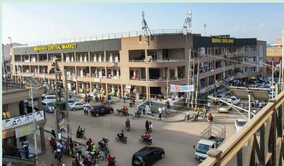
The new Mbarara Central Market, built on 1 acre of land with about 1194 facilities. The new market accommodates 1194 Vendors against 700 vendors that were in the old Market.
